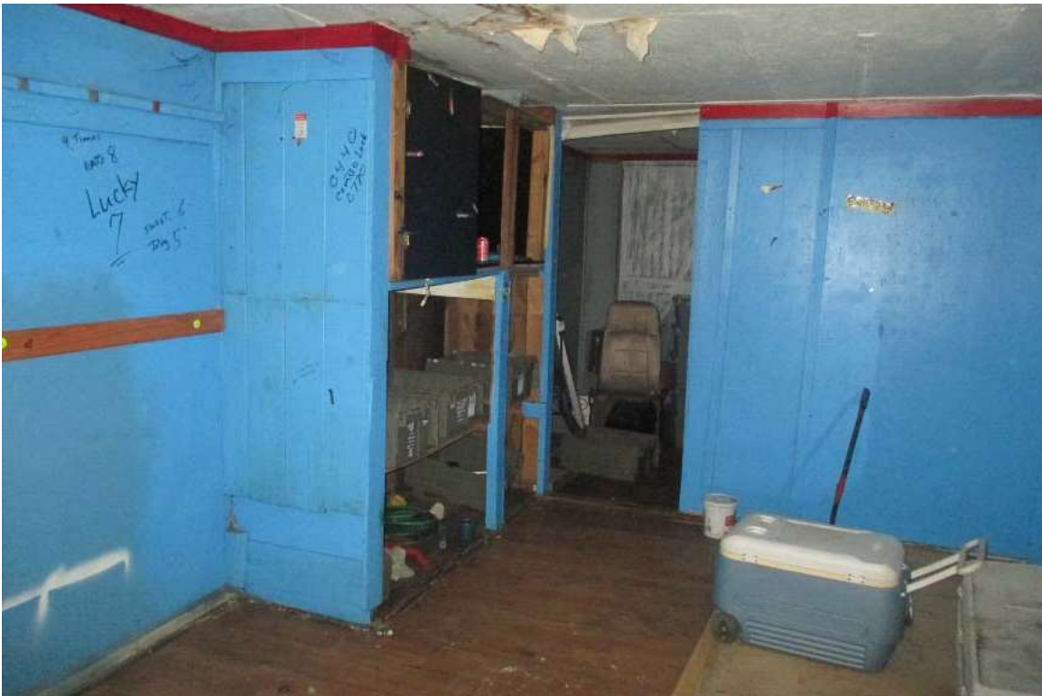
Subject Property - Garage Structure, Interior Spaces
