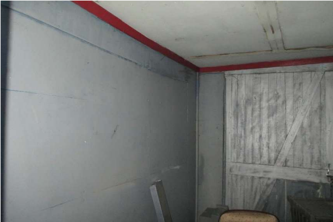
Subject Property - Garage Structure, Interior Spaces
