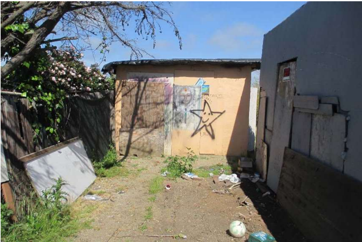
Subject Property - Garage Structure
