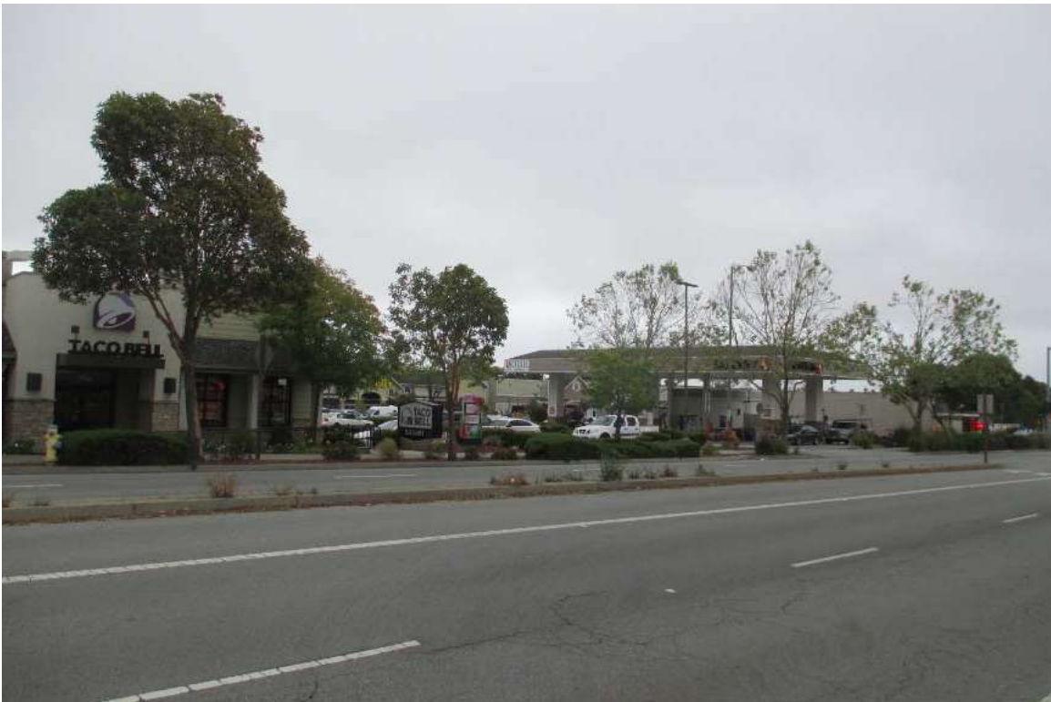
Site Vicinity - Car Wash Located to the Southeast of the Subject Site
