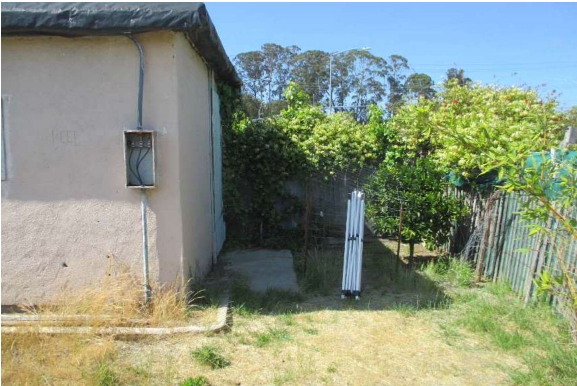
Subject Property - Garage Structure
