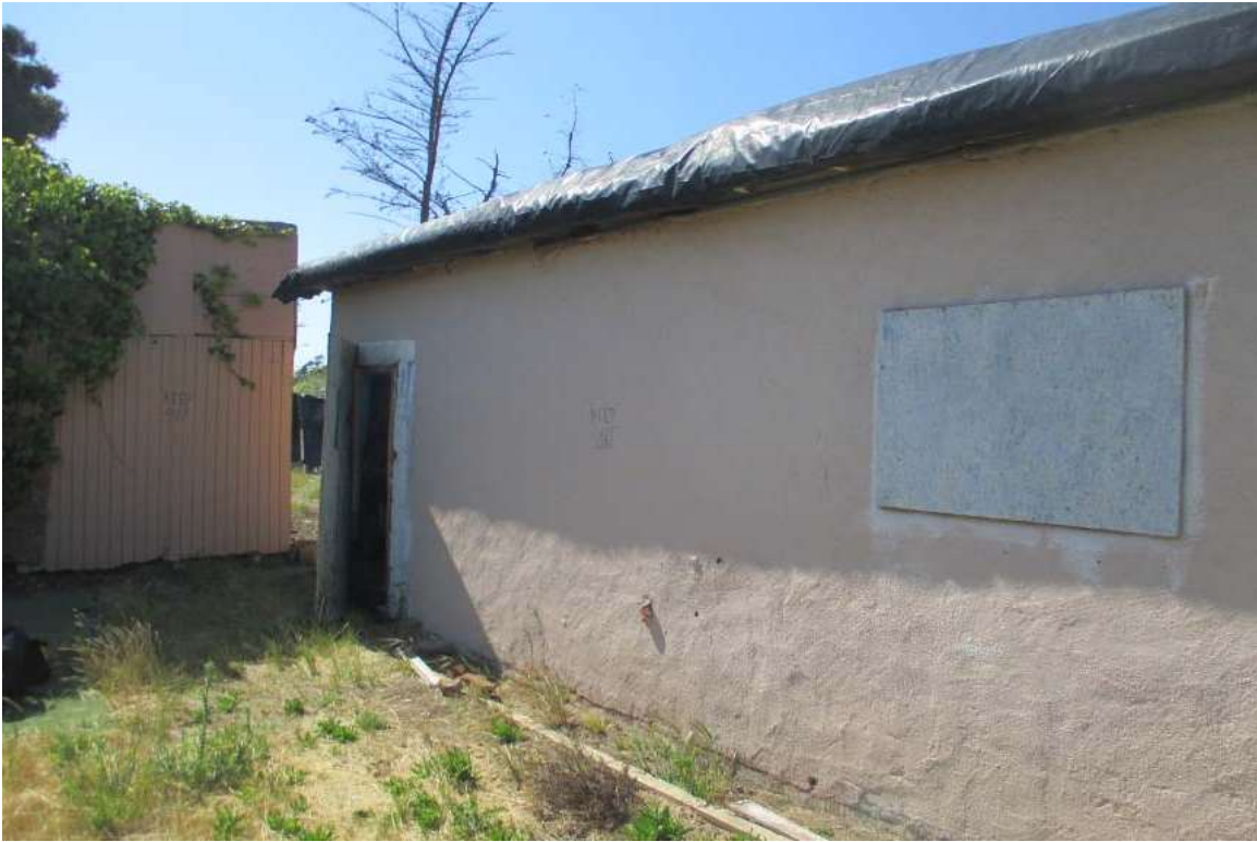
Subject Property - Garage Structure
